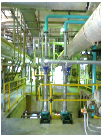
Fig.3 Water Ejectors mounted in site
