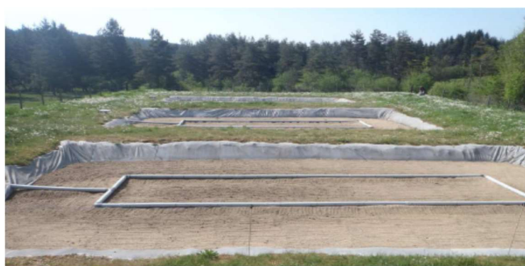
Figure 4 The territorial distribution of the extensive infiltration-percolation basins systems in France and aspects from one of these extensive systems [7]
