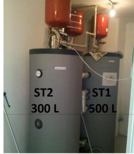
Fig.3 Picture representing the storage tanks
