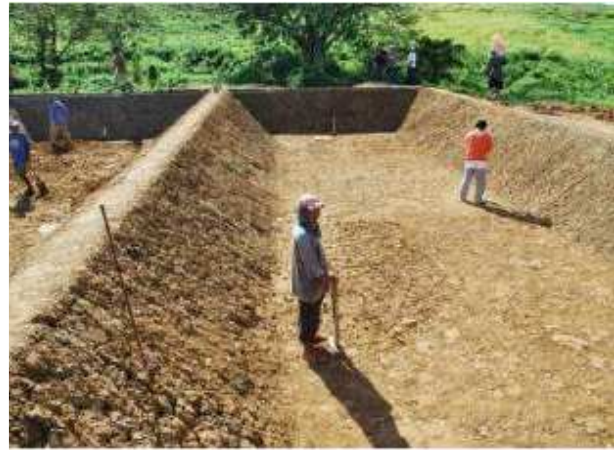
Figure 11: Vertical flow vegetation filter under construction in Bayawan City, Philippines [7]
