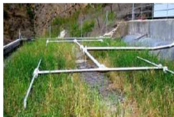
Figure 9: Distribution pipes for wastewater in French System in Albondon, Spain [8]
