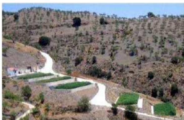
Figure 8: “French System” constructed to treat wastewater from Albondon, Spain [8]
