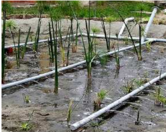
Figure 10: Vertical flow vegetation filter under construction in Lima, Peru [7]
