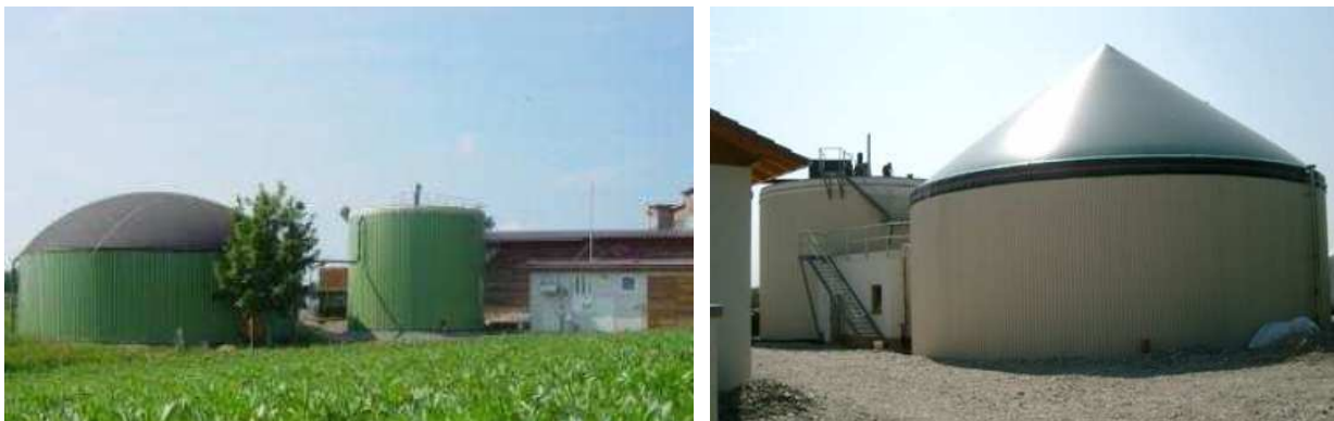
Figure 5: Vertical digesters built in Germany
