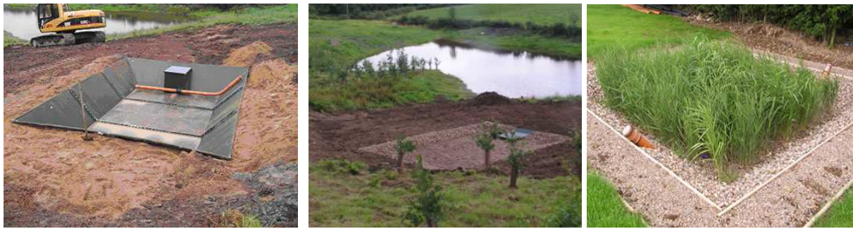
Figure 3: The construction of a horizontal flow vegetation filter in Ireland [5]
