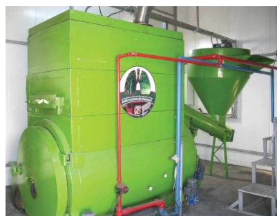
Hot water boiler of 450 kW
