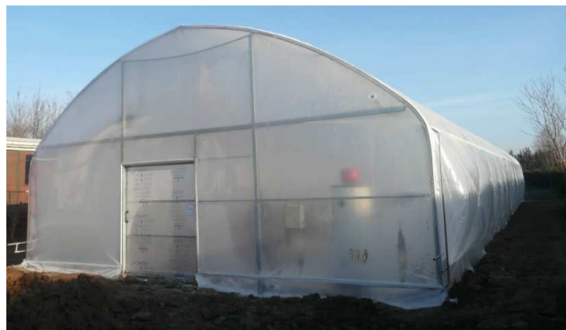
Figure 4: Solar with vertical gothic walls
