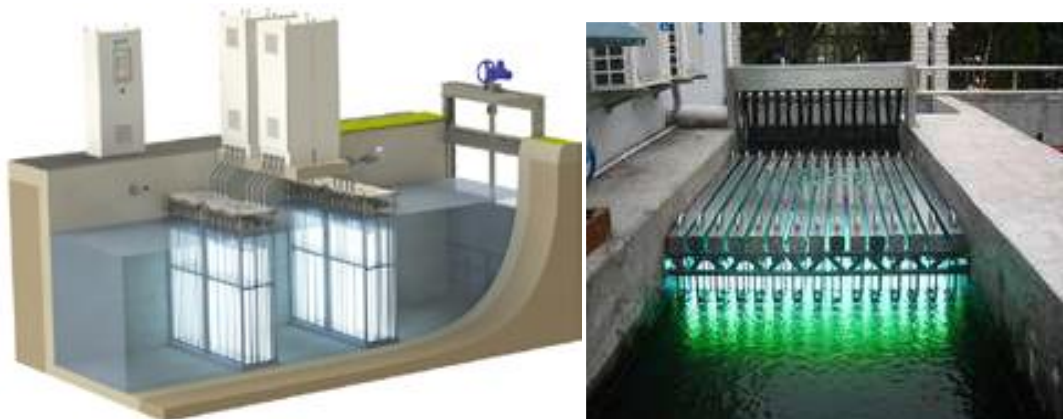
Figure 2: A UV disinfection system [12]
