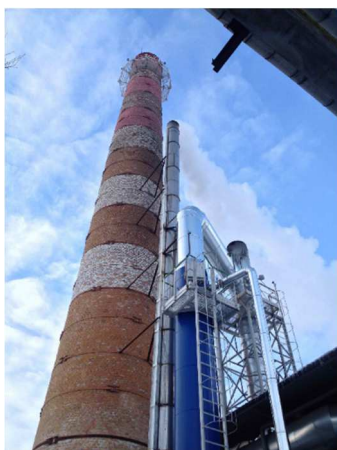
Figure 1: Economizer Enerstena CEB 1000 in biomass boiler house in Boryspil Airport
