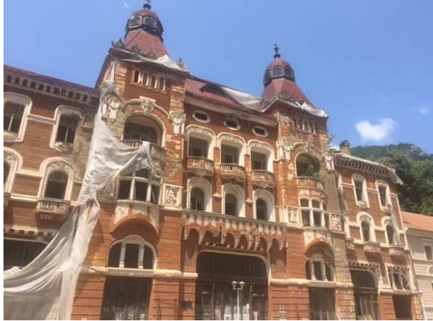
Figure 1: External view of the analyzed enclosure
